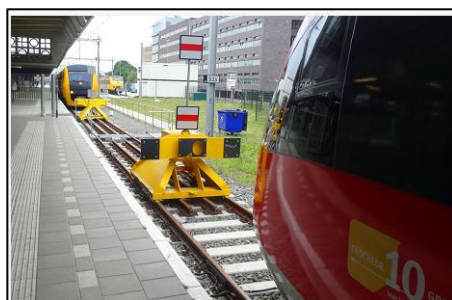
Figure 51: The bump blocks at Enschede station
